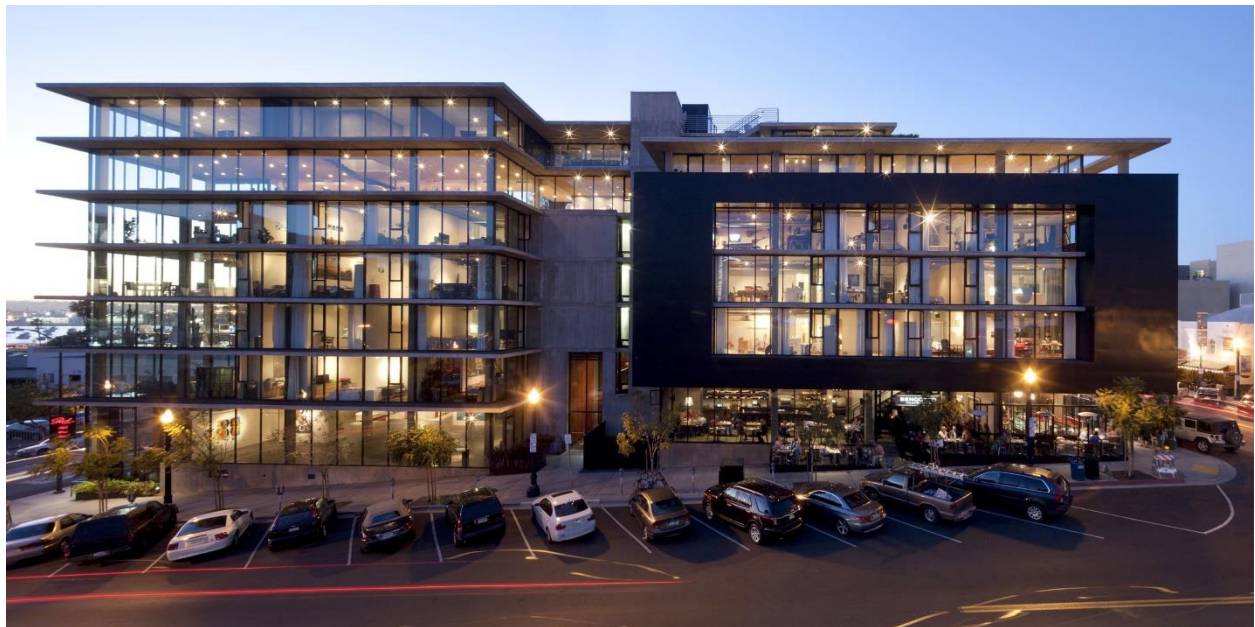
Mid-Rise Residential Mixed-Use Building
